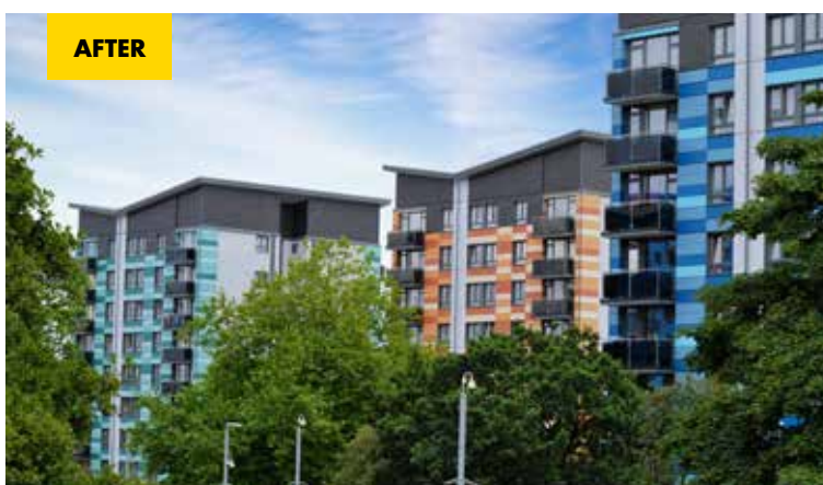
RECLADDING CHARLEMONT FARM ESTATE, UK.
